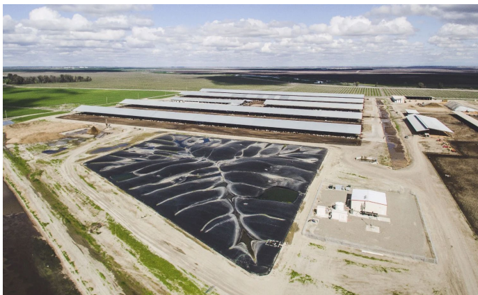
The covered lagoon manure digester creating renewable energy from cow manure, Open Sky Ranch, Riverdale, California
